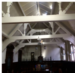
Recreated police court, first floor above cell block
