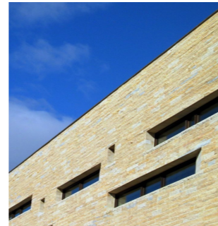
Stone external wall - City & County Museum, Lincoln
